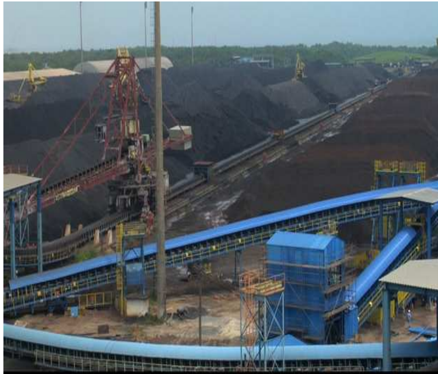
Iron Ore Loading System
